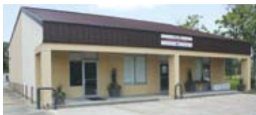
City of Central Municipal Services Center
